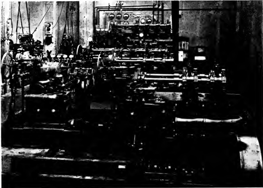
A group of "Kind" engines on the testing stand in the shops at Turin, Italy. These fine Diesels have found a wide use both for mercantile and naval uses.
